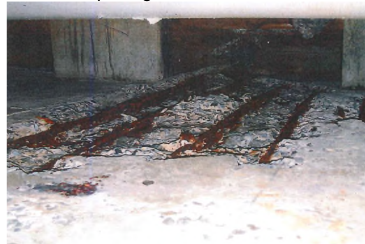
Spalling under concourse
