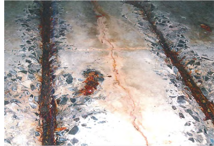
Spalling under concourse
