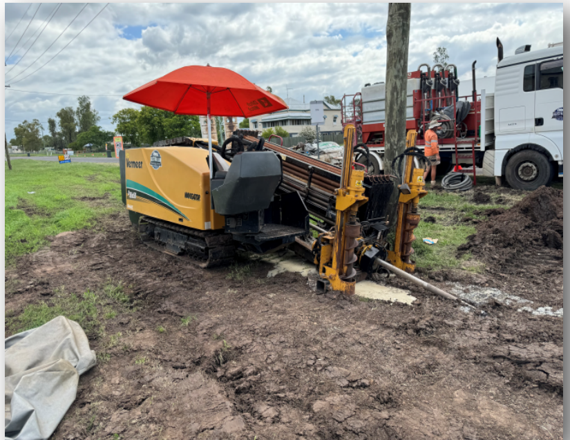
Horizontal Directional Drilling under Warrego Highway at Warra
