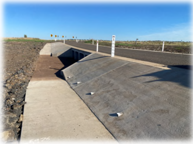
Kleinschmidts Road — Culvert Install Complete
