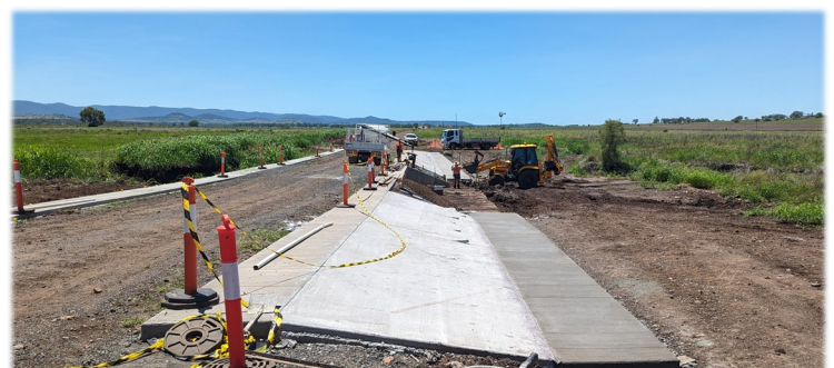
Kleinschmidts Road—Culvert Wingwalls installation
