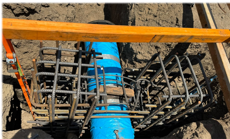
Dalby Water Supply Upgrade - Pipeline Stage 1 - Thrust Block Pre-pour and Dalby WTP Connection
