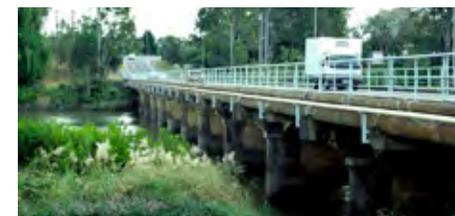
**Lamington Bridge**, Maryborough, was constructed in 1895-1896 as a low-level bridge to withstand regular flooding in the Mary River. Designed by Queensland Government Architect and Engineer for Bridges AB Brady in 1893, it is technologically innovative as one of the earliest concrete bridges in Australia.
