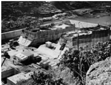
Construction of Somerset Dam
