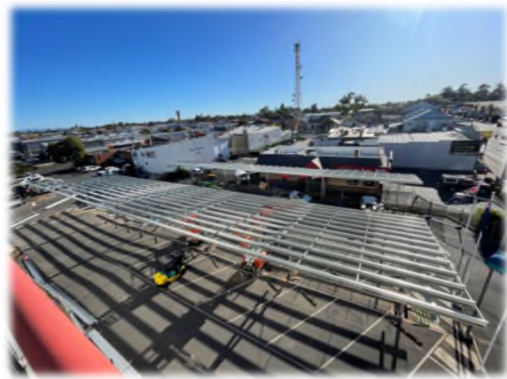
30 Marble Street Installation Construction of Carpark Structure and Solar Panels
