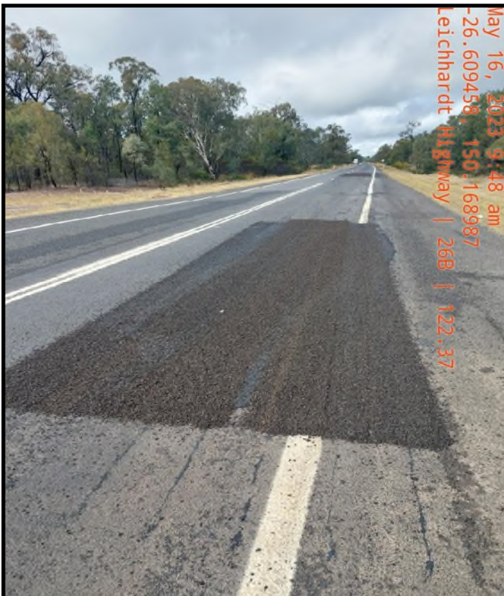
Leichardt Hwy Pavement Repairs
