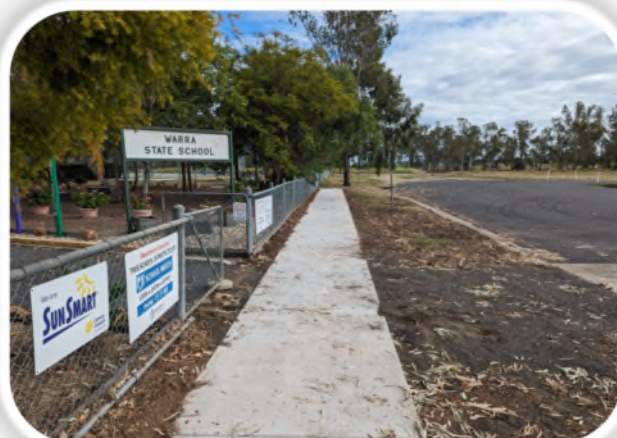
Warra State School New Footpath
