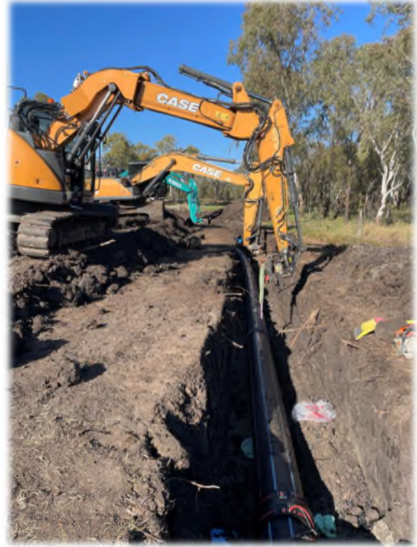
Dalby Water Supply Upgrade - Pipeline Stage 1 Installation of Pipe through Enveloper under Moonie Hwy at WTP
