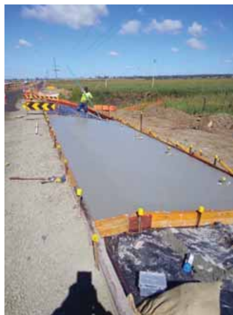
Batter protection under construction
