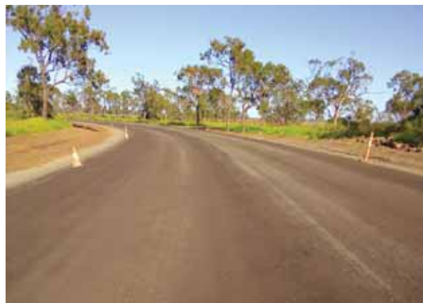
Unbound pavement ready for seal
