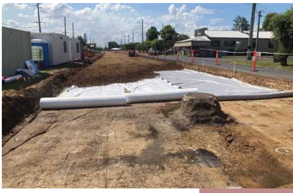
Glenmore Road - subgrade and placement of subbase layer on geofabric
