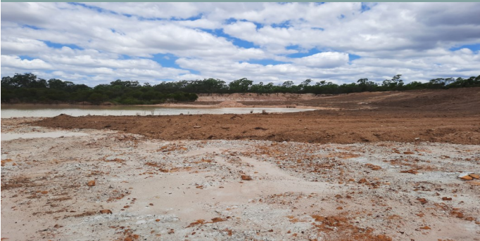
Rehabilitation commenced at Keys Pit
