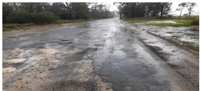
Section of Broadwater Road to be upgraded by Arrow Energy
