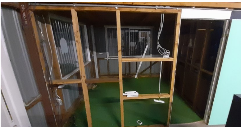
Chinchilla SES Facility Upgrades in Progress
