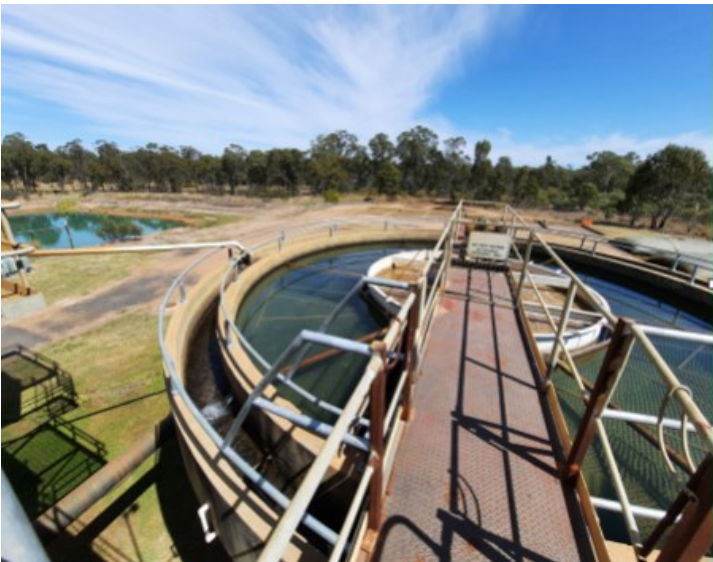
New hand rails installed at Miles WTP
