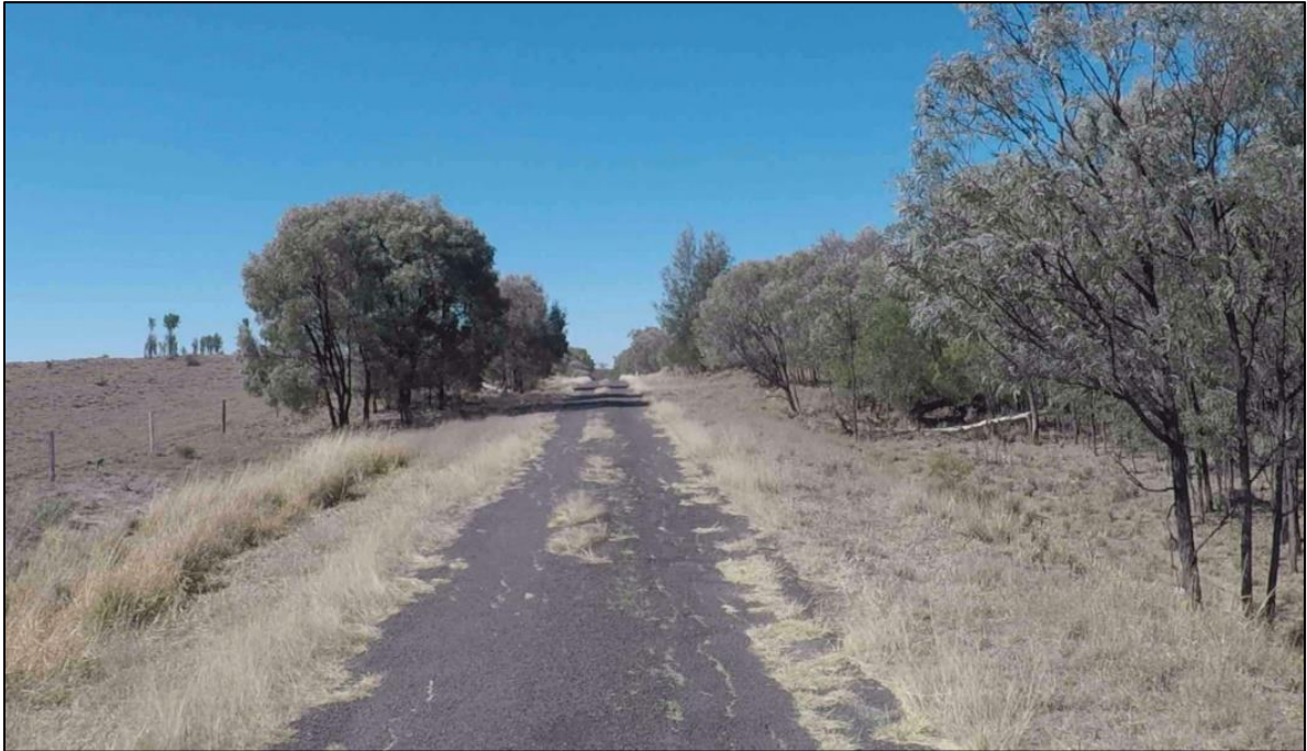
Figure 2 - Juandah Creek Road RACAS Imagery (taken Sept 2017)
