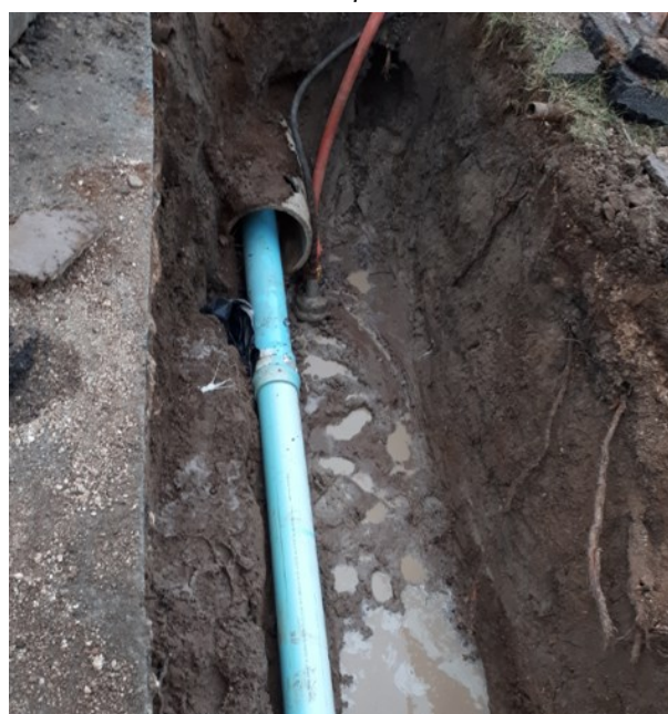
Tara Water Main Repair in Rail Corridor
