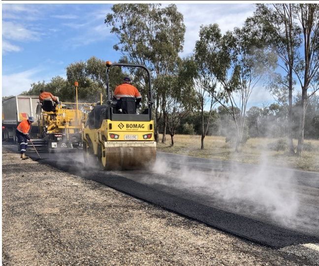
Asphalt repairs on Surat—Developmental Road
