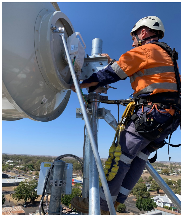
Microwave Equipment Replacement at Jandowae
