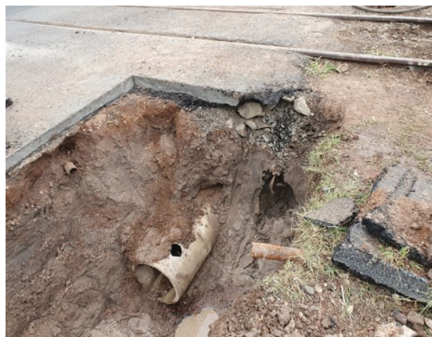
Tara Water Main Repair in Rail Corridor
