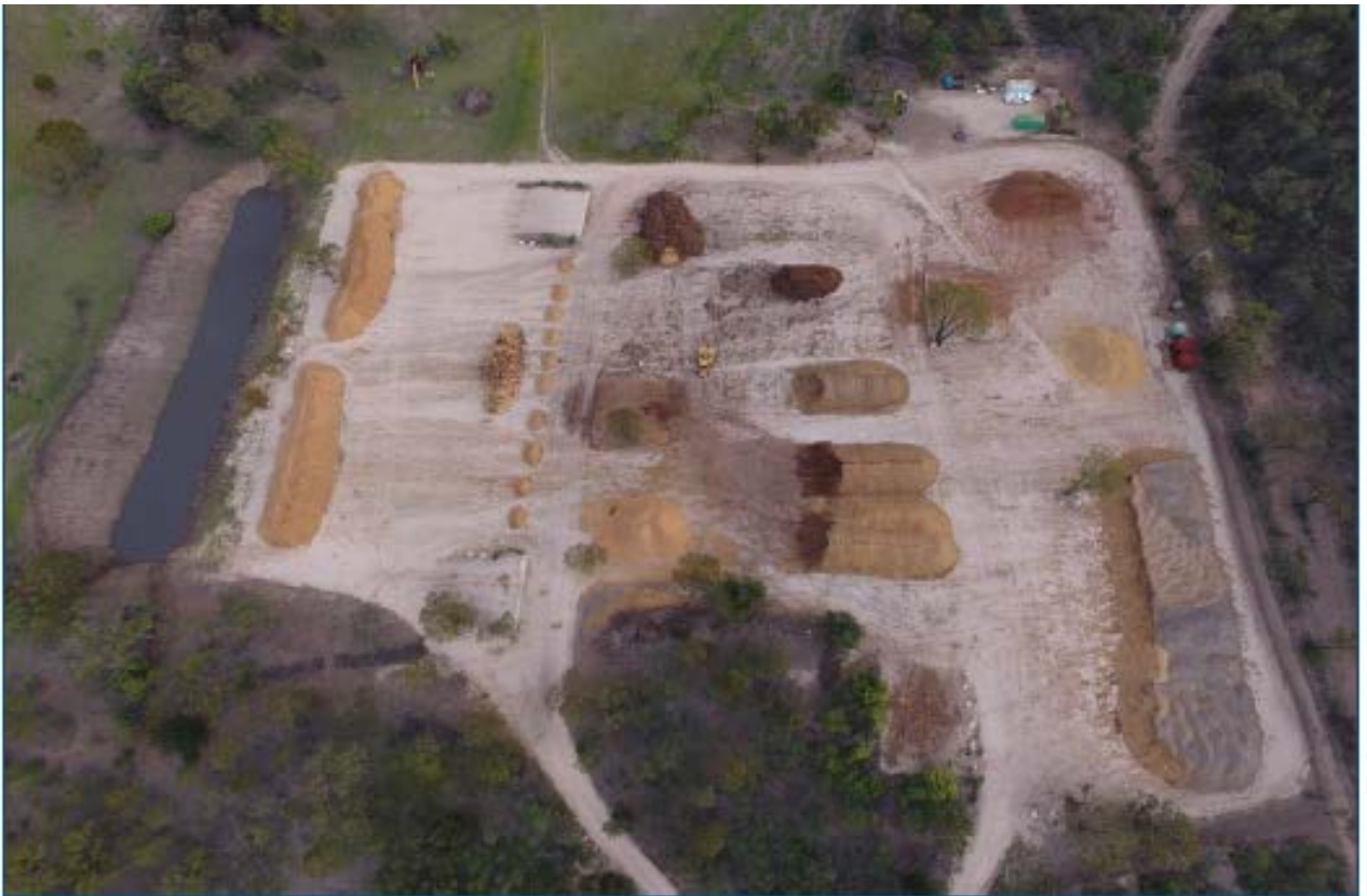
Aerial View of existing Warehouse Hardstand Area
