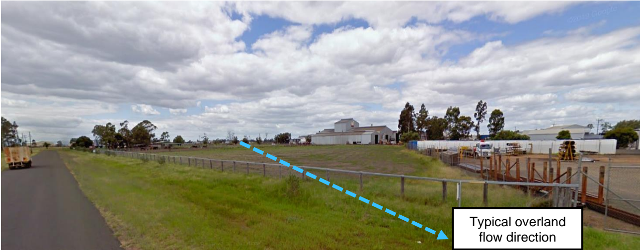
Figure 1-3 Site as seen from Volker Street, looking North-East (Google Street View)
