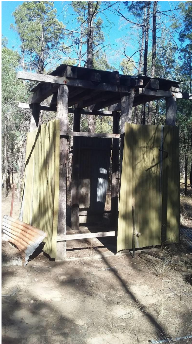
Figure 3 - Water Tank Tower & Showers
