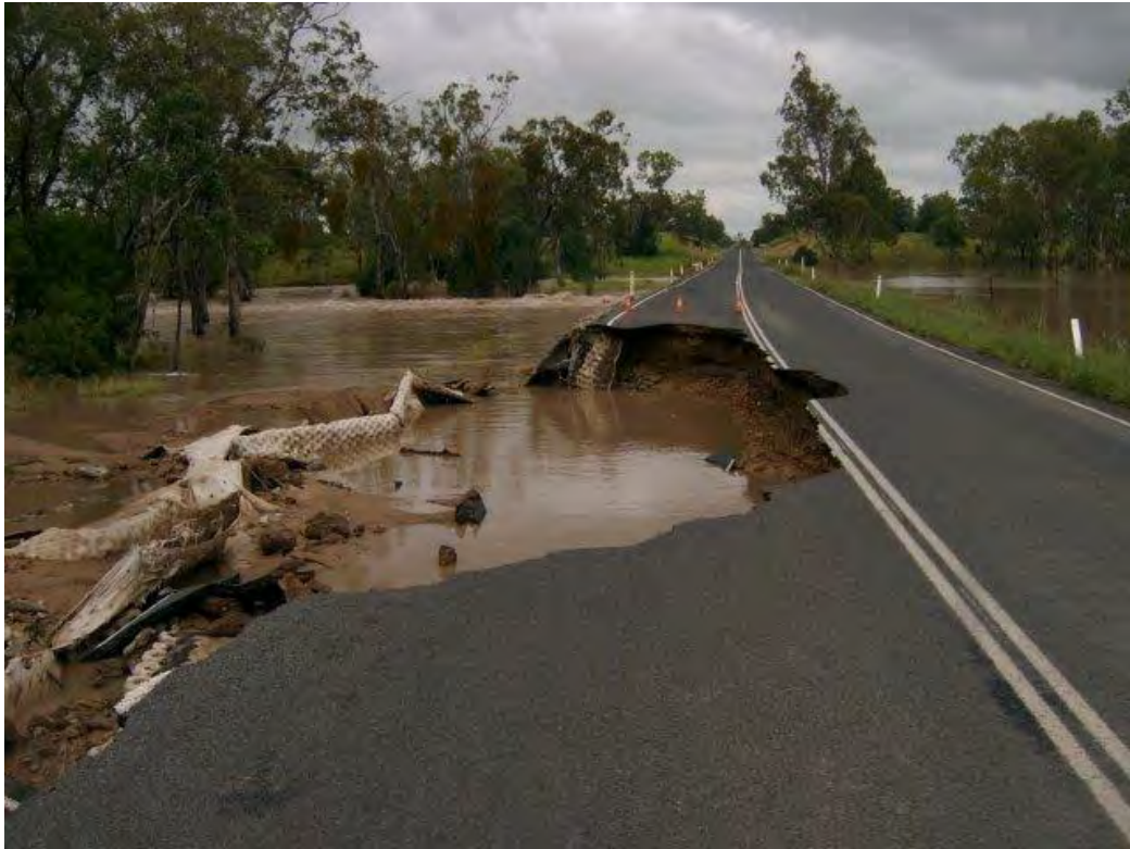
Figure 3-7 Flood Damage to Leichhardt Highway North of Wandoan
